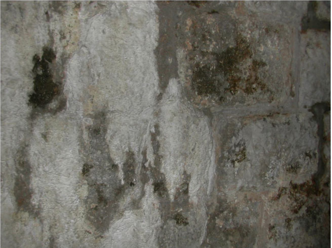
Fig. 4: outcomes of carbonation processes, namely incrustations , on limestone wall blocks, Dubrovnik (Croatia).
