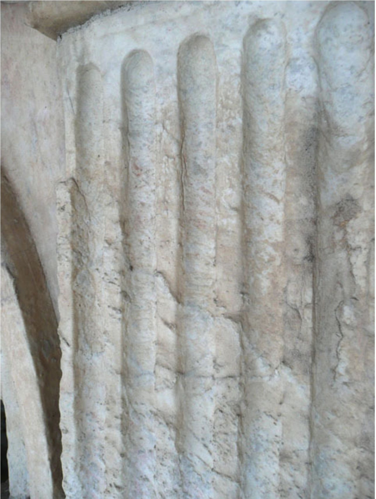
Fig. 8: wind driven erosion of a white marble pillar's surface, Florence Cathedral dome (Italy).
