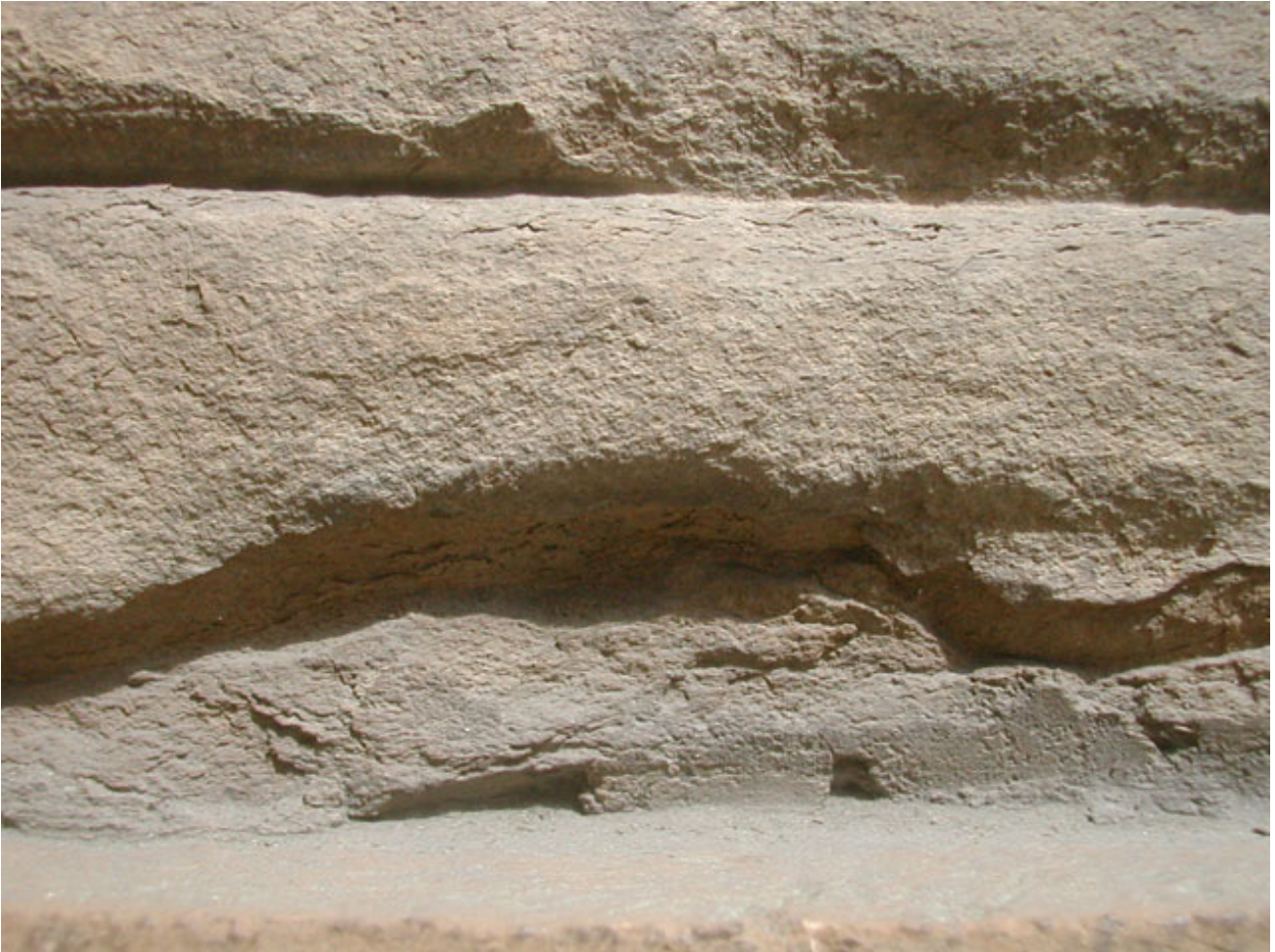
Fig. 5: effects of argillification on a long exposed XV cent. sandstone , Florence (Italy).
