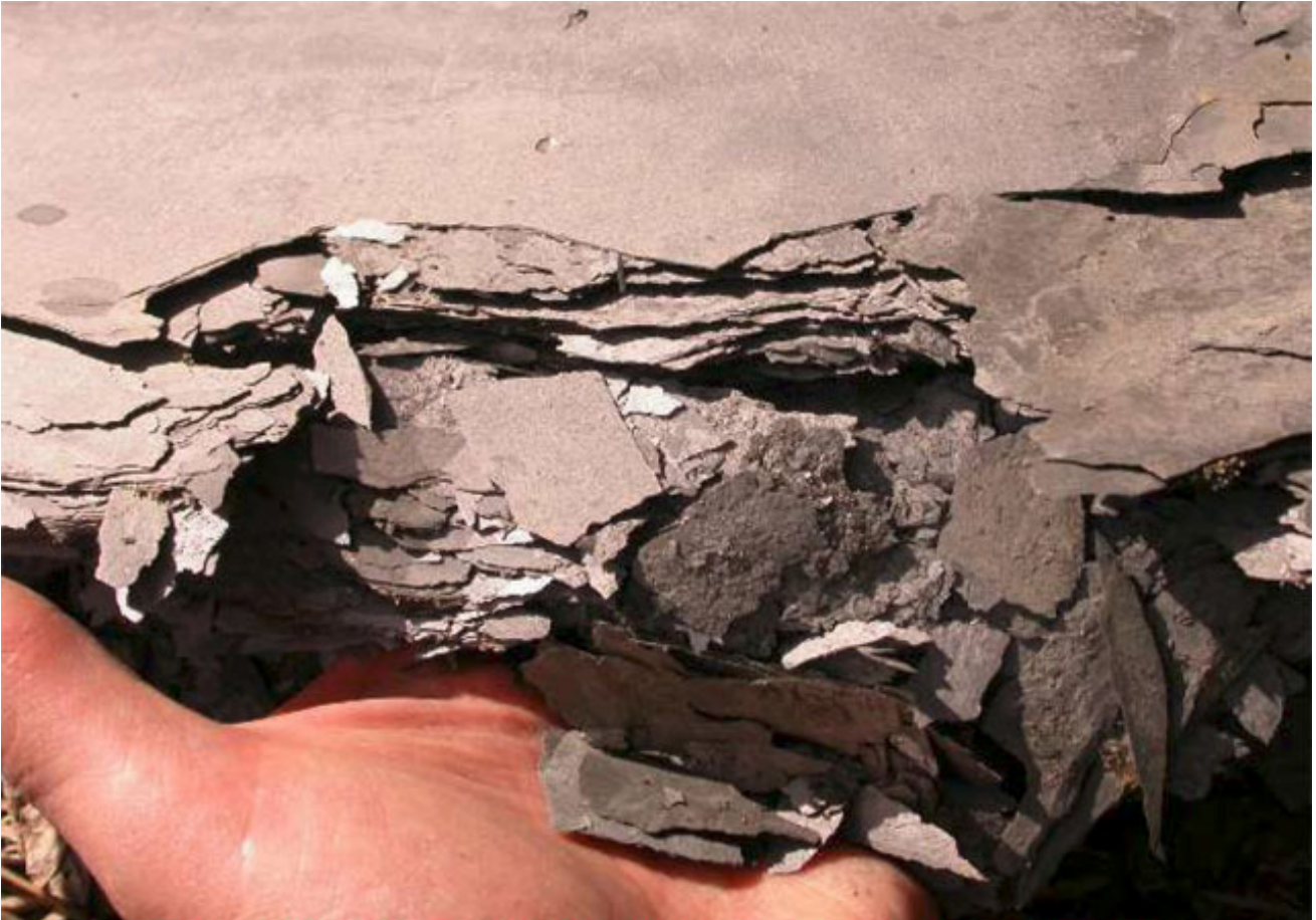
Fig. 9: weathered slate softening and delaminating, Pennsylvania (USA).
