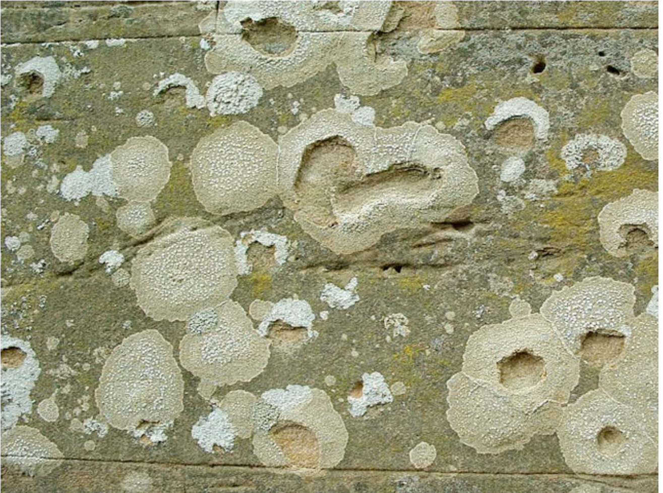
Fig. 6: surface of well tooled sandstone blocks covered and deteriorated by lichens' growth, Scotland (Great Britain).
