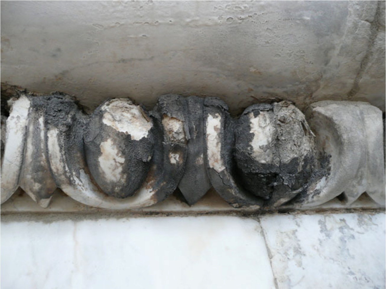
Fig. 10: “egg and darts” decoration affected by sulphatation and consequent black crusts formation, Florence Cathedral dome (Italy).
