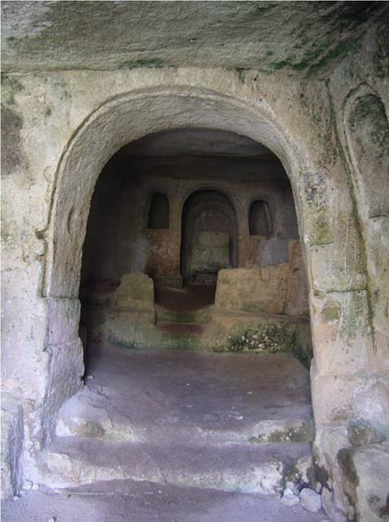
Fig. 7: the growing of cyanobacteria on the surface of a rock cut monument, Matera (Italy).
